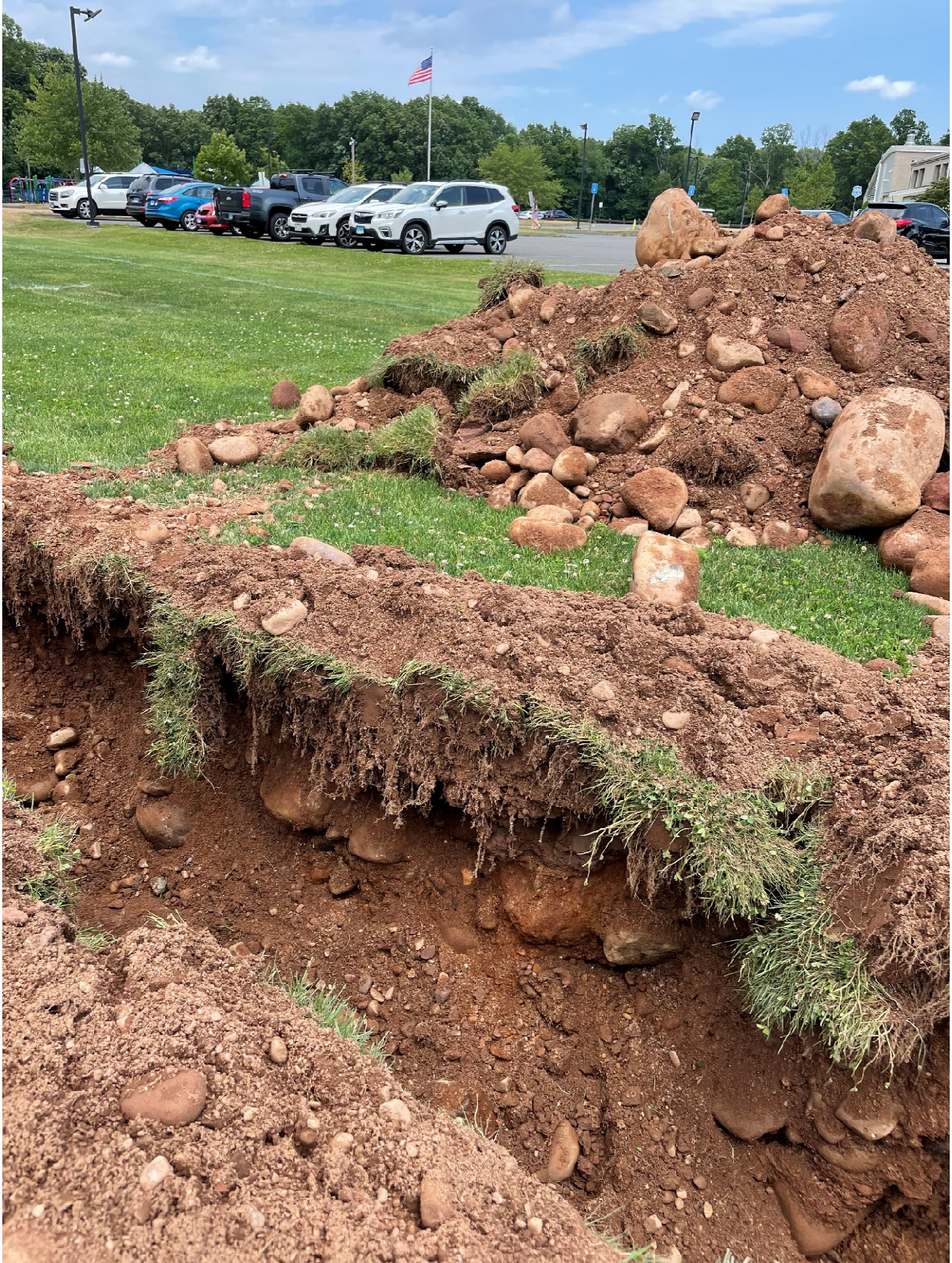
Photo 3: TP-32, located along the eastern side of the athletic fields
